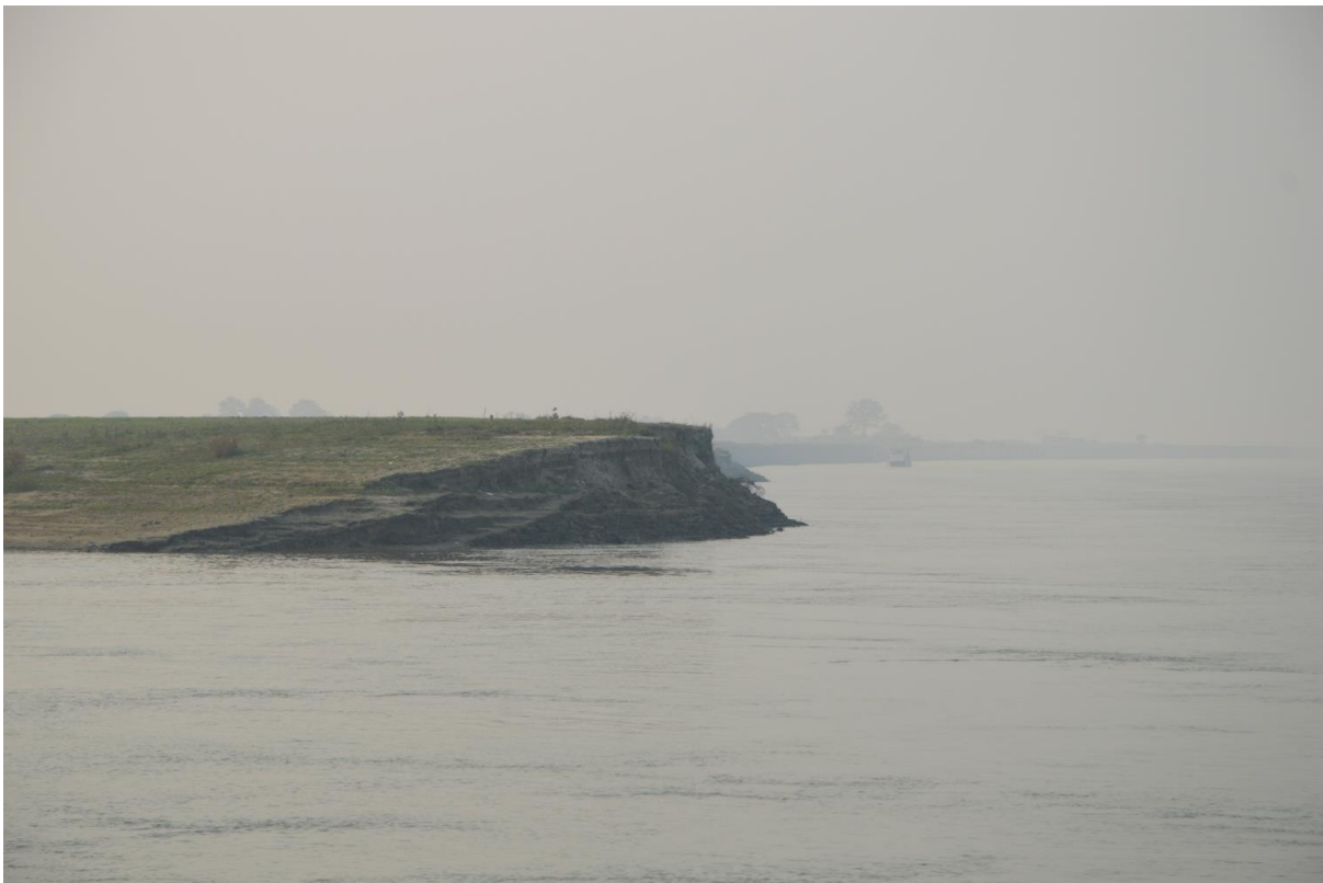
Image 26 : Erosion Prone Site Near Sahibganj Town
